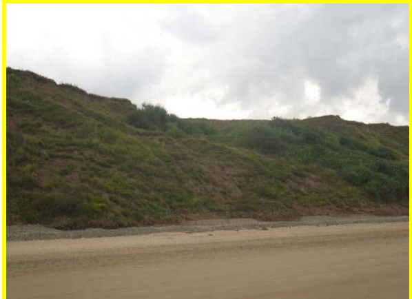
MU29/AN Toe erosion on an otherwise vegetated slope (Locally Active).
