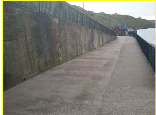
Promenade ramp above seawall (Asset Ref. 1221D901D0802C04)
