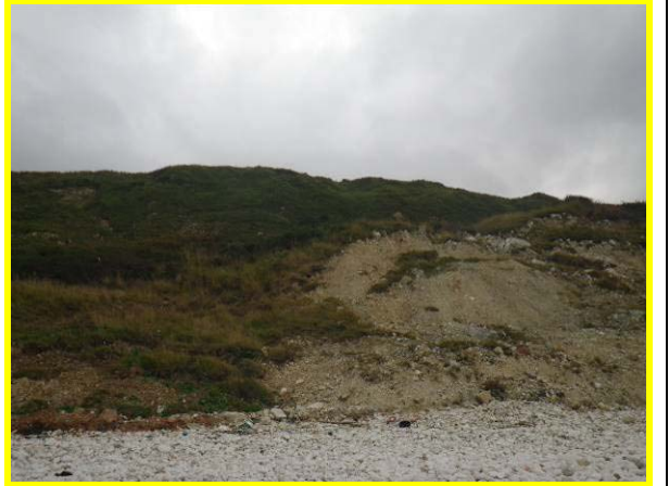
MU29/CI Actively eroding cliff toe (Locally Active)
