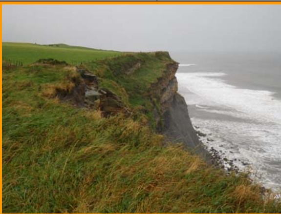
MU13/5 The cliff is showing signs of erosion in the lower half of the face (Partly Active).
