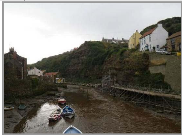
(No unit) - Further up Staithes Beck a rockfall occurred in the cliffs during February 2012. The site was remediated in September 2012.
