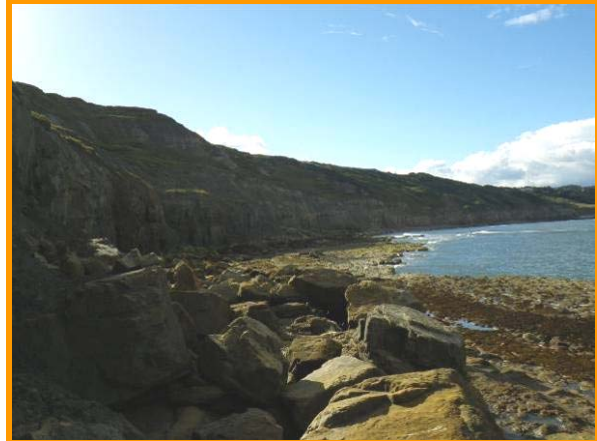
MU23/D1 failed blocks at the toe of the cliff (Partly Active)
