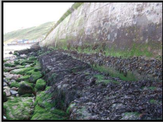
Washout of joints in slabs from wave overtopping (Asset Ref. 1221D901D0802C03)
