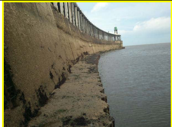
General view of west outer breakwater (Asset Ref. 1221D901D0803C01)
