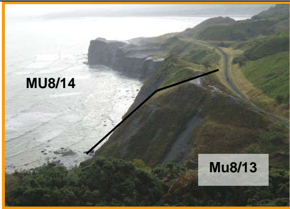
MU8/13 and MU8/14 Erosion at the toe of the units causes instability to propagate up the face of the cliff (Partly Active) (approx. extents shown).
