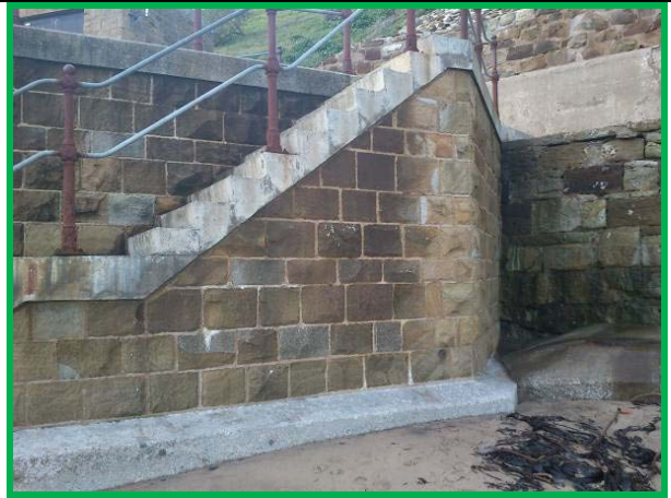
Seawall around the pumping station (Asset Ref. 1221D901D0601C07)
