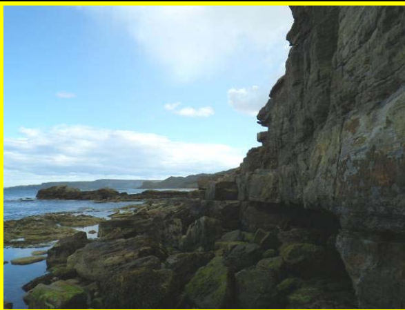
MU23/D2 The failed material is evident on the shore (Partly Active)
