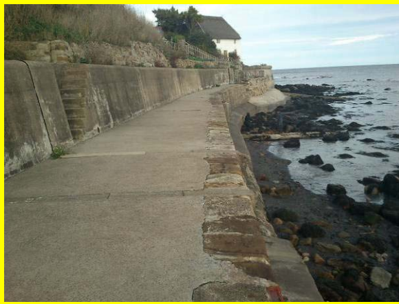
Overview of wall (Asset Ref. 1221D901D0601C03)
