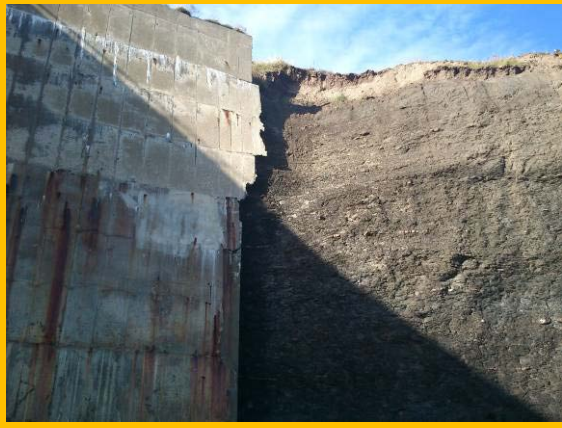
Large vertical wall at Robin Hood's Bay (Asset Ref. 1221D901D1003C02)
