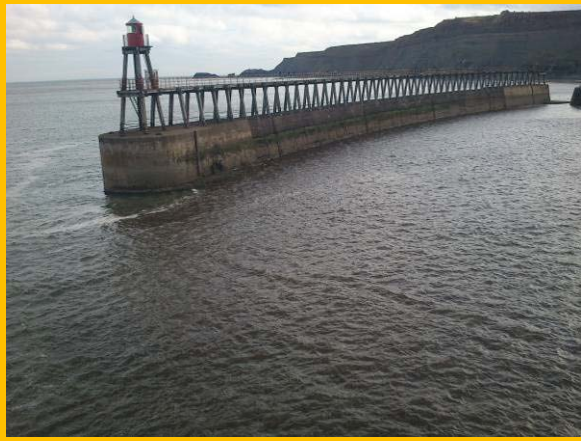
General view of outer east breakwater extension arm, (Asset Ref. 1221D901D0803C04)
