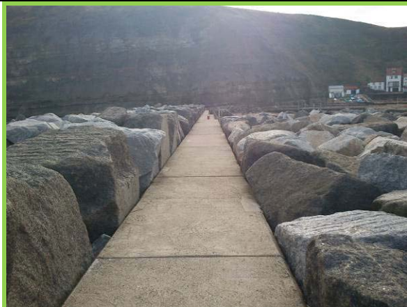
South breakwater promenade and rock armour (Asset Ref. 1221D901D0403C03)
