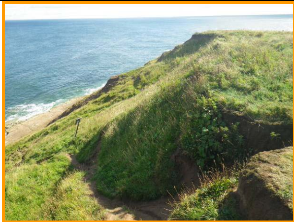
MU27/A Cracking and slumping activity (Partly Active)
