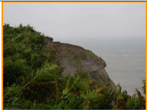
MU15/2 An area of intense erosion (Partly Active)
