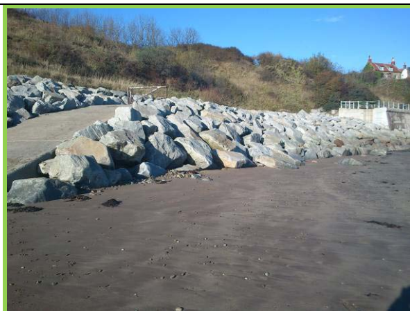
Rock armour and ramp south of Quarter Deck (Asset Ref. 1221D901D1003C09)
