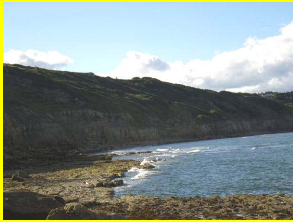
MU23/C Ongoing marine driven erosion is evident on this unit (Locally Active)
