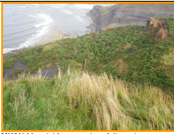
MU8/4 Material from previous failures have stabilised and become vegetated above the level of wave attack (Partly Active)
