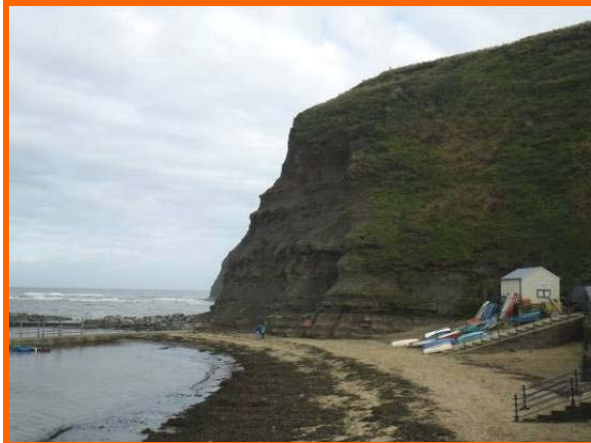
MU4/2 –Vegetated cliff with localised erosion, behind Staithes harbour (Partly Active).
