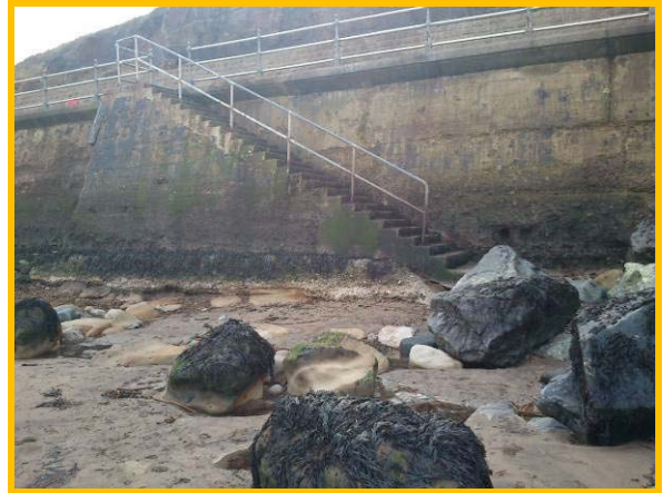
Undermining of wall adjacent to steps - (Asset Ref. 1221D901D0802C03)
