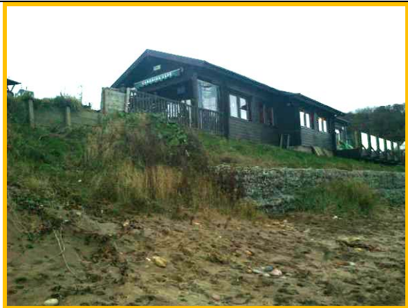
Gabions protecting café at NW end of revetment (Asset Ref. 1221D901D0702C02)
