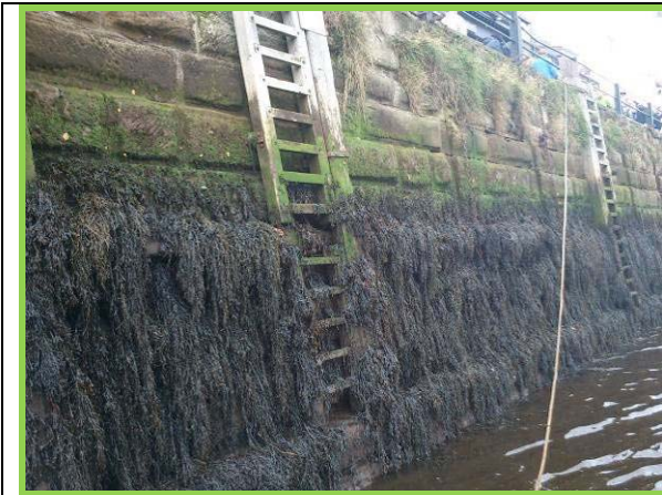
Inner west quay wall near swing bridge, (Asset Ref. 1221D901D0803C07)
