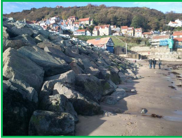
Runswick Bay village rock armour defences (Asset Ref. 1221D901D0602C01)
