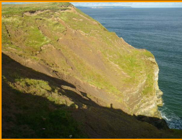
MU27/BB Mass failure of upper layer (Partly Active)
