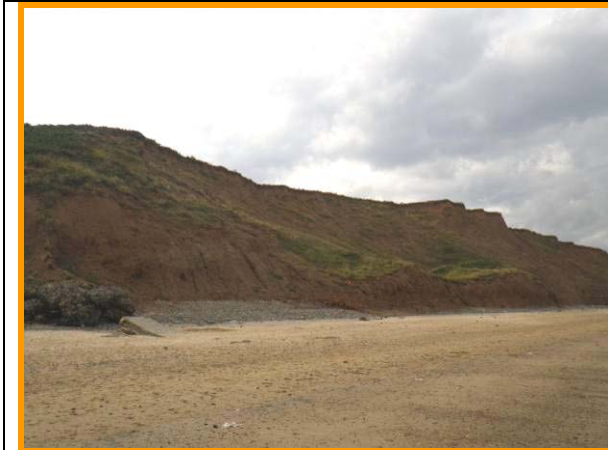
MU29/BE Headscarp and toe erosion (Partly Active).
