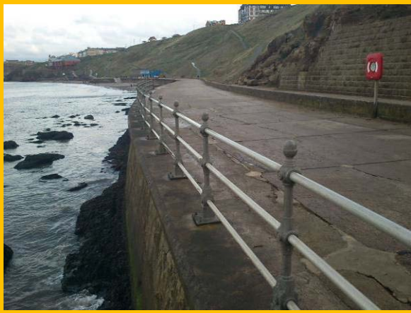
Washout of joints in slabs from wave overtopping (Asset Ref. 1221D901D0802C03)
