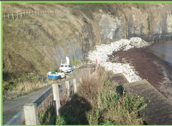
Rock armour at north end of defence system (Asset Ref. 1221D901D1003C02)
