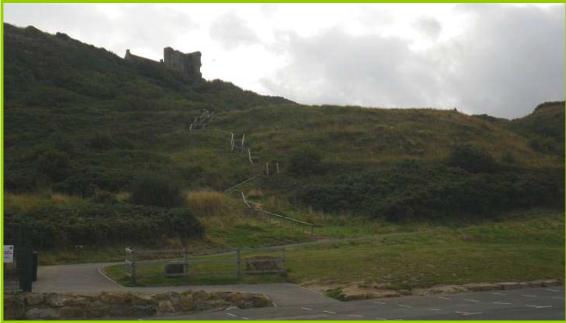
MU21/1 Well jointed hard rock has a thick cover of vegetation (Inactive).
