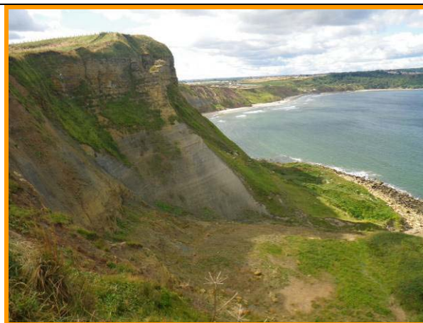
MU25/V Upper part of active mudslide system (Partly Active)
