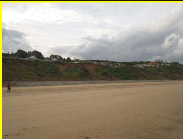
MU29/AR Continuing mudslide activity and toe erosion at Flat Cliffs (Locally Active).
