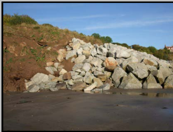
Southern extent of rock armour - photo from 2009 inspection (Asset Ref. 1221D901D1003C07)
