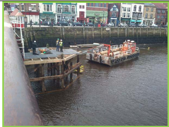
Repairs underway to swing bridge fendering
