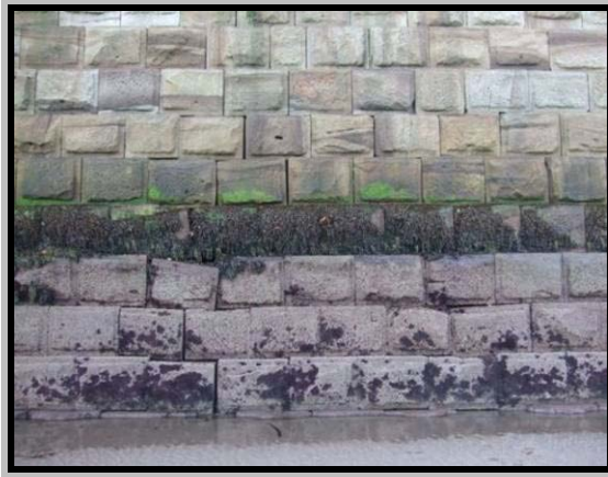
Displacement of block work on west side of West Breakwater - left image from 2009, right from 31/10/12 (Asset Ref. 1221D901D0803C02)
