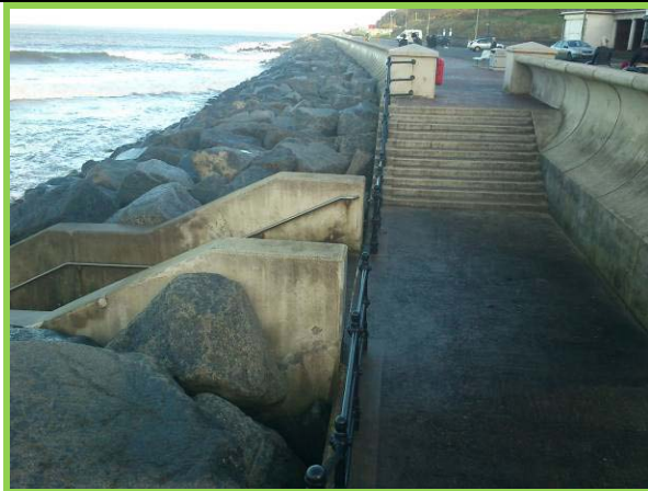
Overview of rock armour with raised crest wall (Asset Refs. 1221D901D1202C03)
