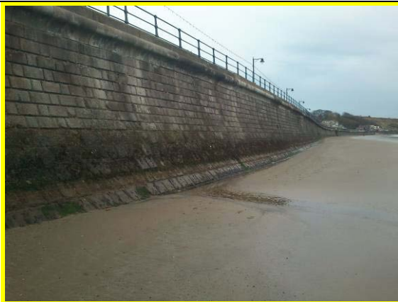
General view of wall looking north. (Asset Ref. 1221D901D1602C03)
