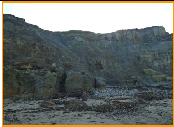
MU23/B Recent failure of the cliff (Partly Active)
