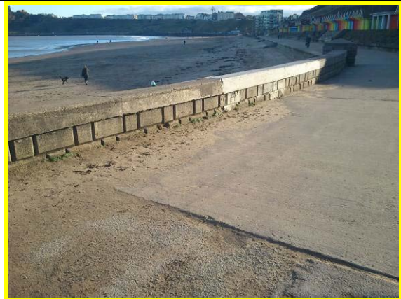
Recent repairs to low crest wall at promontory. Asset Ref. 1221D901D1201C04
