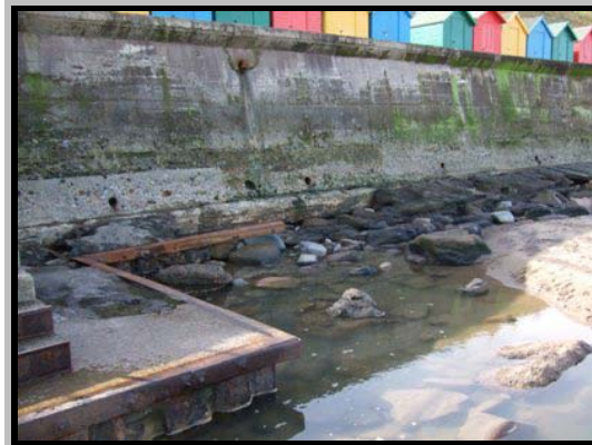
Photos of exposed and damaged toe (Asset Ref. 1221D901D0802C03) – From 2009 inspections
