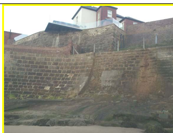
Walls protecting former pumping station (Asset Ref. 1221D901D1402C05)
