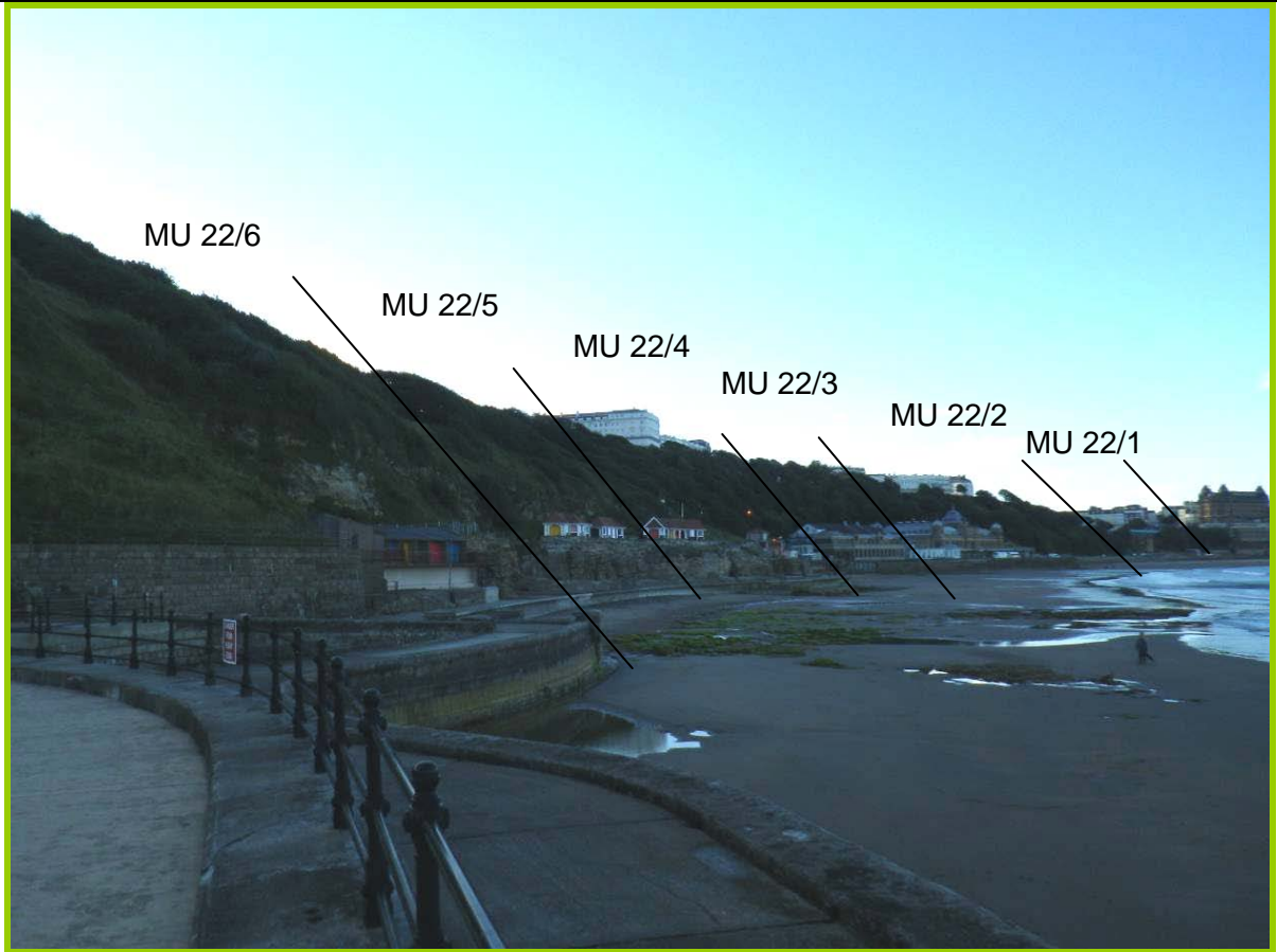
MU22/1 to MU 22/6 Well vegetated slopes with large coastal defences at the toe (Inactive)
