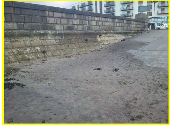
Slipway and sloping wall with splash beam (Asset ref. 1221D901D1201C20)
