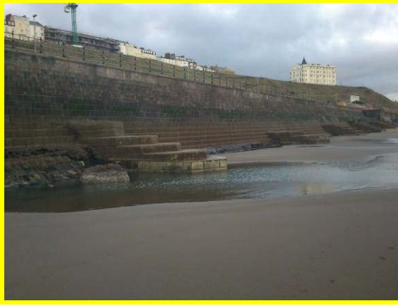
Looking north from south end (Asset Ref. 1221D901D1201C08)
