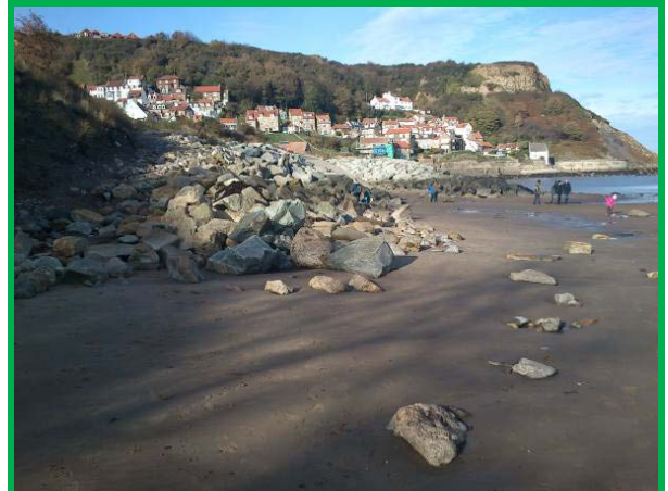
Southern end of Runswick bay rock armour defences (Asset Ref. 1221D901D0602C01)
