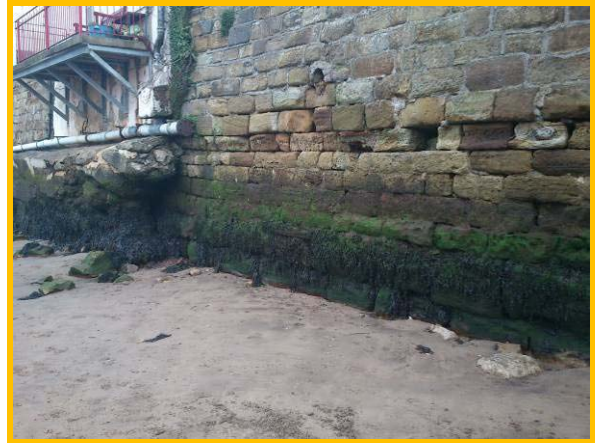
Wall at east side of harbour south of Tate Hill pier (Asset Ref. 1221D901D0803C08)
