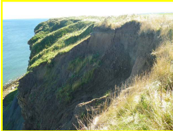
MU25/AD Erosion affecting the top of the cliff (Locally Active).
