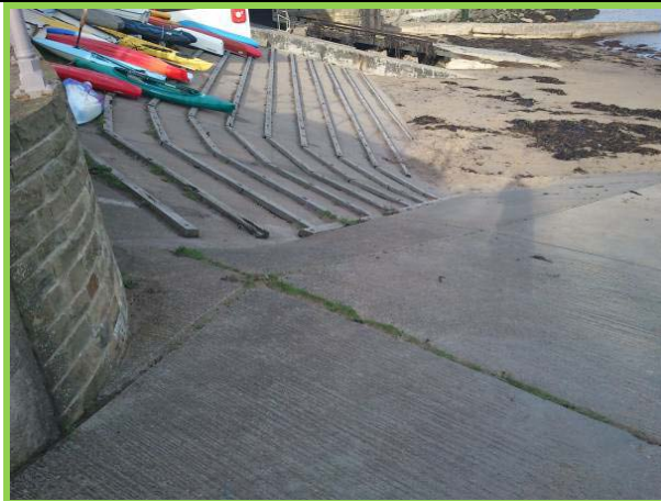
Northern slipway adjacent to the RNLI (Asset Ref. 1221D901D0601C04)
