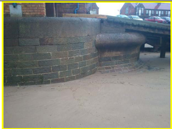
Minimal change to wall since 2009 (Asset Ref. 1221D901D1301C08)
