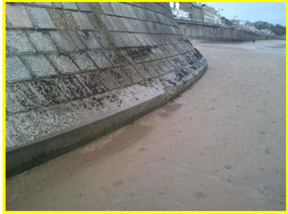
Repaired section of toe with chipped block adjacent. (Asset Ref. 1221D901D1602C04)
