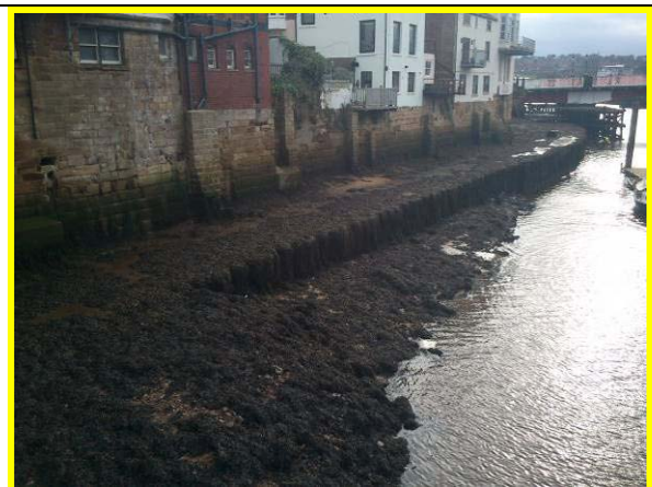
Sheet piling and toe apron protecting property walls (Asset Ref. 1221D901D0803C10)
