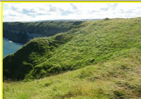
MU26/AG Rockfall evidence at the unit toe (Locally Active)
