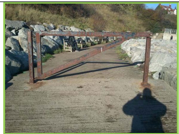
Promenade above rock armour. (Asset Ref. 1221D901D1003C09)
