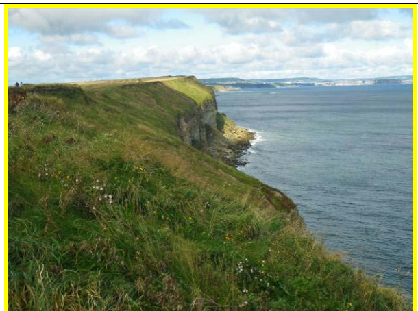
MU26/AX Localised erosion of upper soft till layer (Locally Active)
