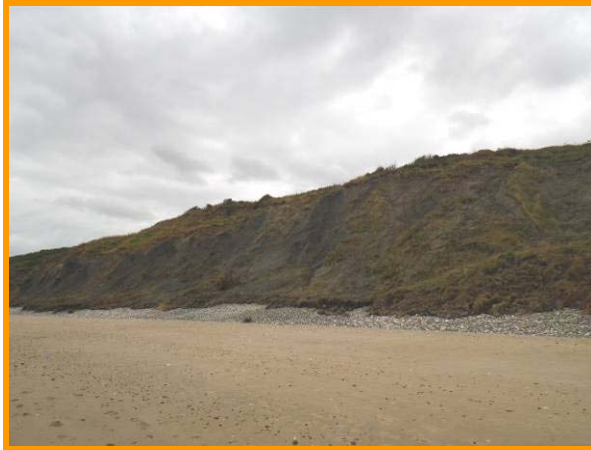
MU29/CC Erosion and mudsliding at Middle Cliff (Partly Active)
