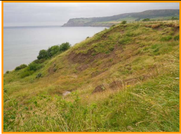
MU17/2 The slope is showing evidence of ground movement (Partly Active).
