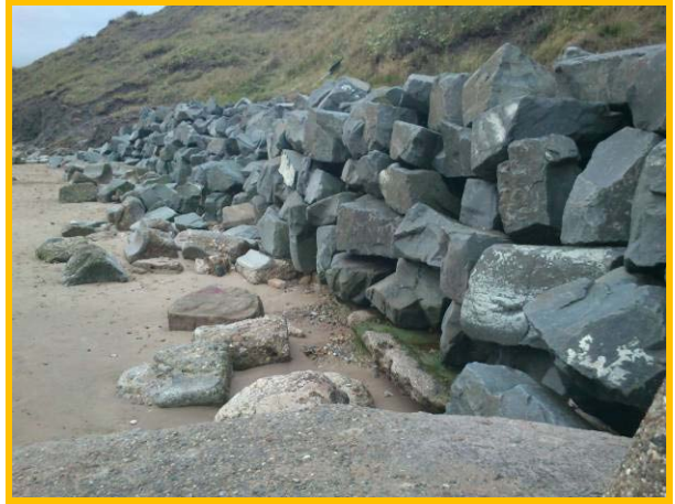
Rock revetment with gabion baskets beneath. 09/11/2012. (Asset Ref. 1221D901D1602C02)
