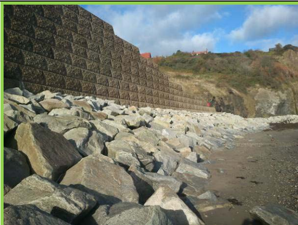
Sea wall with rock armour toe constructed in 2001 (Asset Ref. 1221D901D1003C01)
