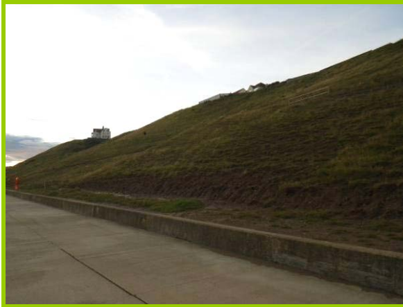
MU11/1 Regraded, stabilised slopes (Inactive)
