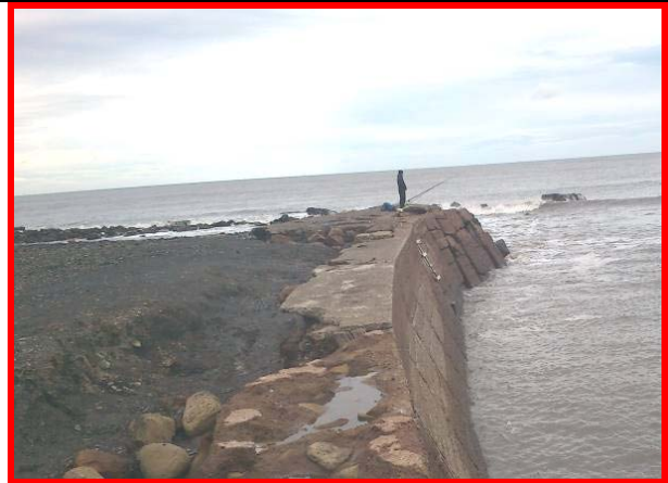
View of breakwater 30/10/2012 (Asset Ref. 1221D901D0502C01)
