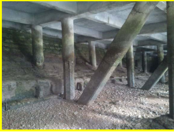
The original quay wall beneath the newer concrete jetty (Asset Ref. 1221D901D1301C06)
