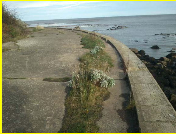
Promenade on top of northern seawall, 30/10/2012 (Asset Ref. 1221D901D0601C01)
