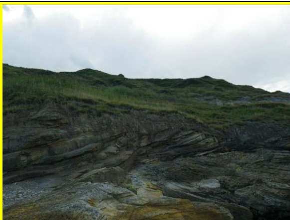
MU23/E Vegetation and localised erosion (Locally Active)
