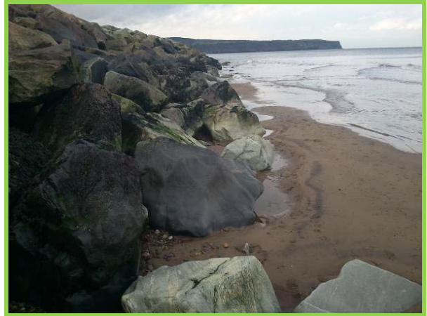
Rock armour in good condition (Asset Ref. 1221D901D0801C01)
