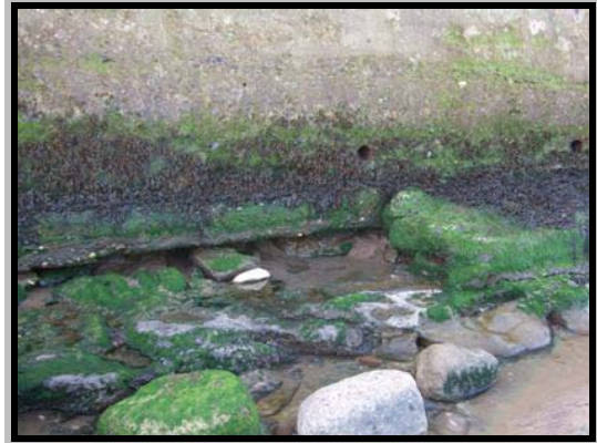
Undermining of wall adjacent to steps - (Asset Ref. 1221D901D0802C03)
