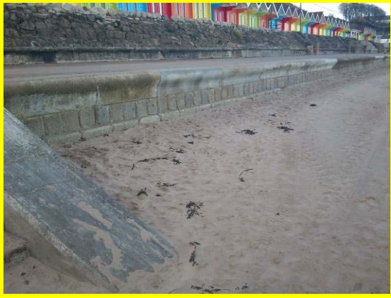
High beach levels, repairs to capping beam holding. (Asset Ref. 1221D901D1201C12)
