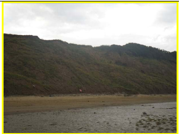
MU29/AB Eroding toe and sliding mid-slope (Locally Active)
