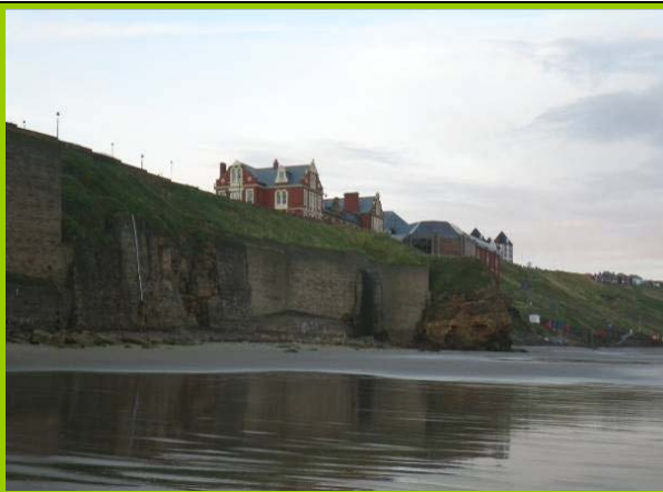
MU11/3 Defended slopes with little evidence of recent activity (Inactive)
