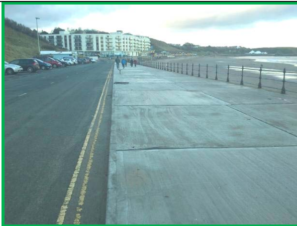
Recently replaced promenade slabs (Asset Ref. 1221D901D1201C07)
