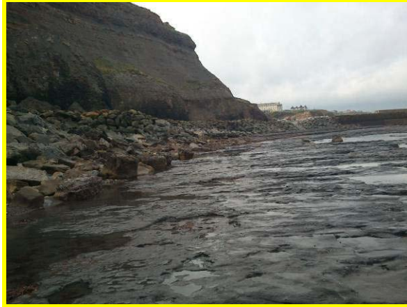
Rock armour protection to toe of Abbey Cliff (Asset Ref. 1221D901D0803C05)
