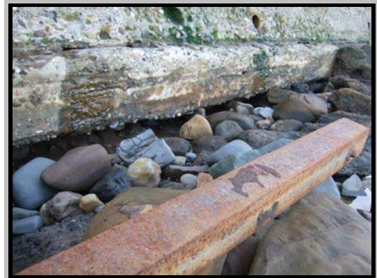
Photos of exposed and damaged toe (Asset Ref. 1221D901D0802C03) – From 2009 inspections
