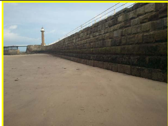
General view of West breakwater (Asset Ref. 1221D901D0803C04)
