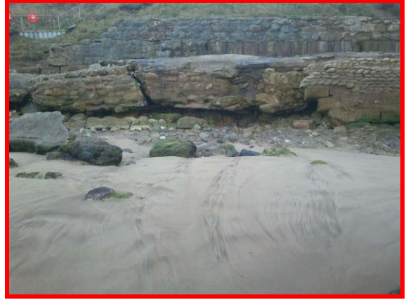
South end defence of the pumping station (Asset Ref. 1221D901D1402C04)
