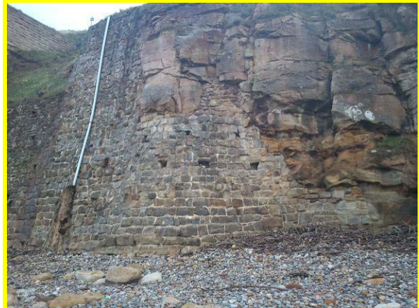
Cliff protected with blockwork, (Asset Refs. 1221D901D0802C09)
