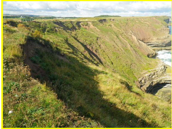
MU27/BE The vegetated slopes are showing signs of slippage and ongoing coastal erosion (Locally Active)
